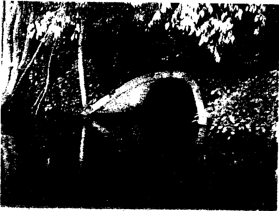
Outfall in the northwest corner
